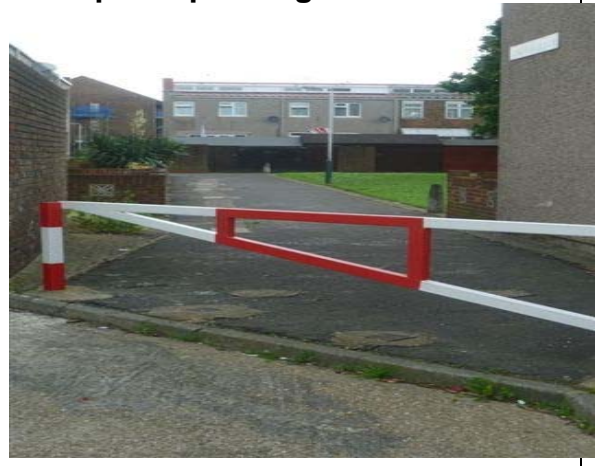
Example of painting work:
